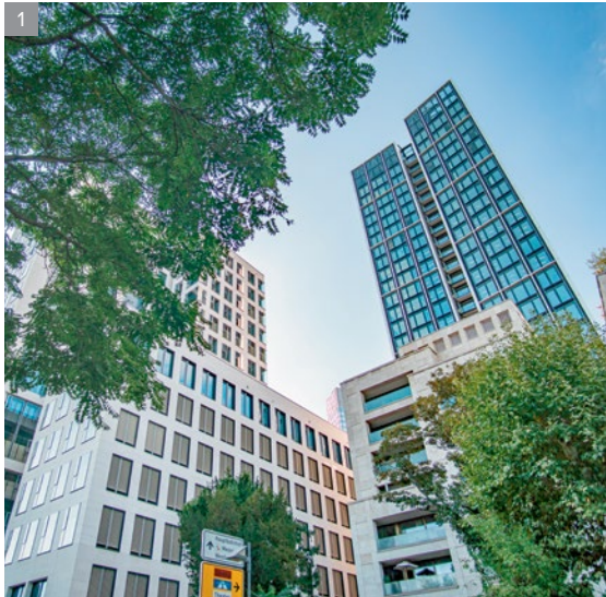
1 WinX Tower Frankfurt/Main, Germany Architect: KSP Jürgen Engel Architects DGNB Platinum certificate 9 elevators 6 high speed elevators
