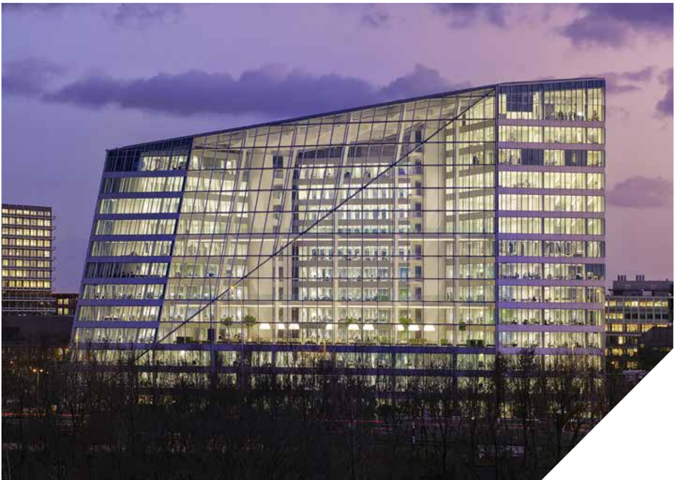
The Edge - The Netherlands - Mini DBE - Awarded with the BREEAM Award for Offices New Construction
