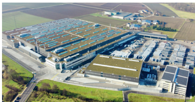
Plant 3 in Cleebronn
