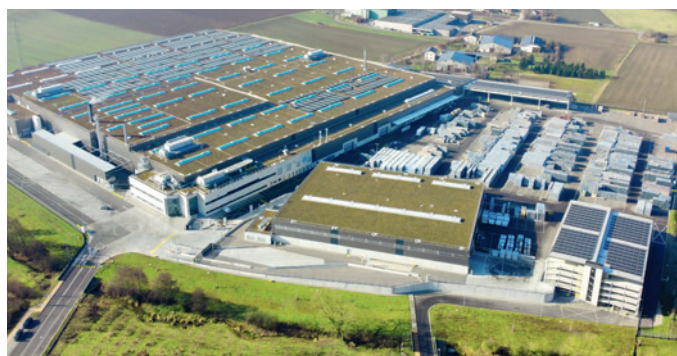
Plant 3 in Cleebronn
