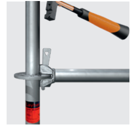
Hammer down the wedge to provide a non-positive connection (Use 500 g metal hammer until the blow bounces off).
