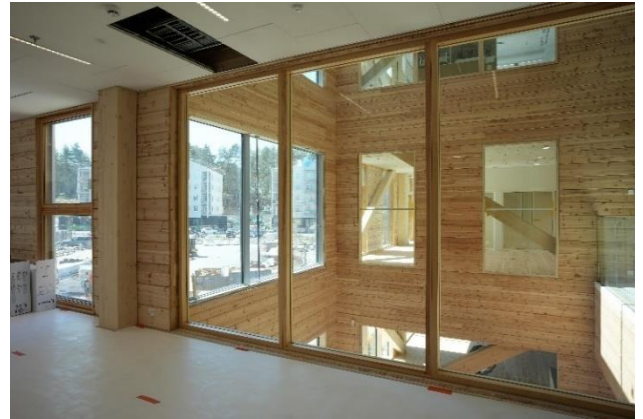
Wood framed glass walls and full glass walls with wood profile
