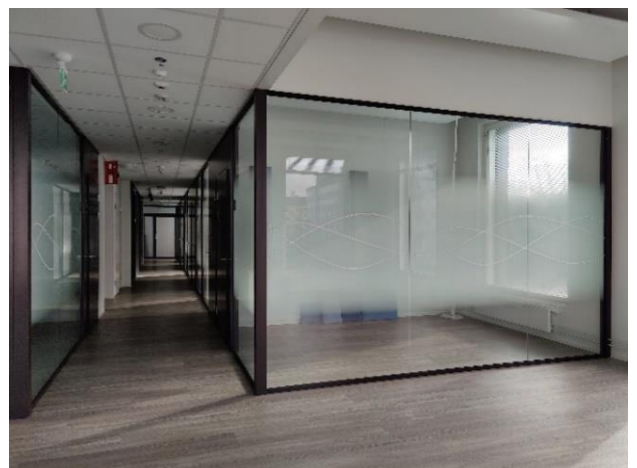
Full glass walls with aluminium profile
