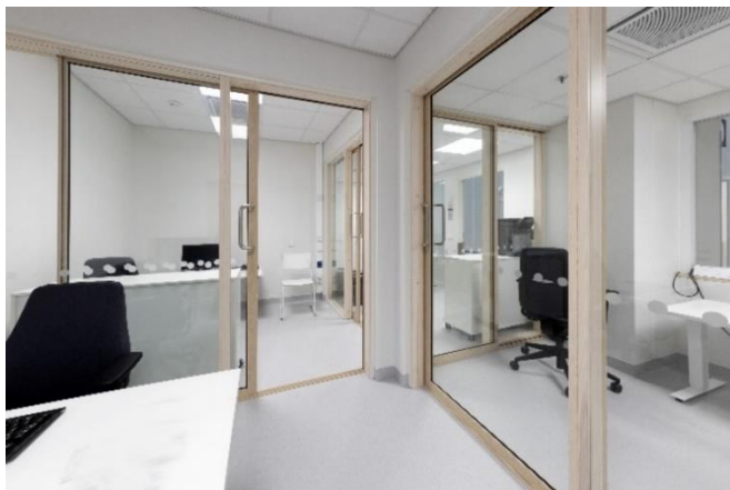
Aluminium framed glass walls
